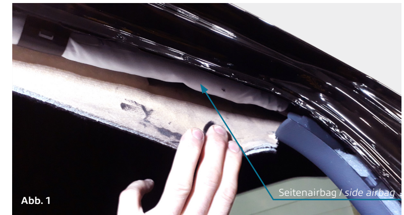
Abb. 1 Dachhimmel heruntergezogen / roof sky pulled down to access bolts
